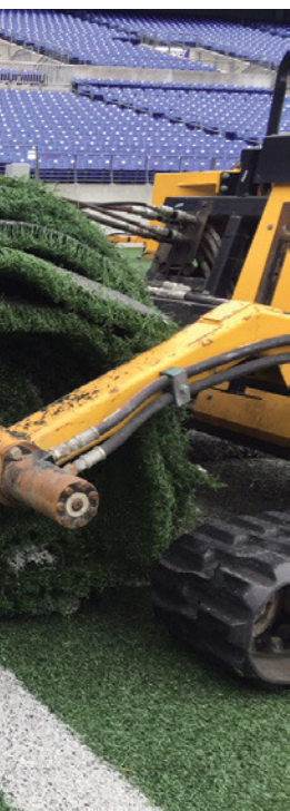
By May, crews were installing the irrigation system at M&T Bank Stadium and sodding with Tifway 419 bermudagrass, a more robust variety than the turfgrass used there in 1998 and the gold standard for football fields where bermudagrass is the turf of choice.
