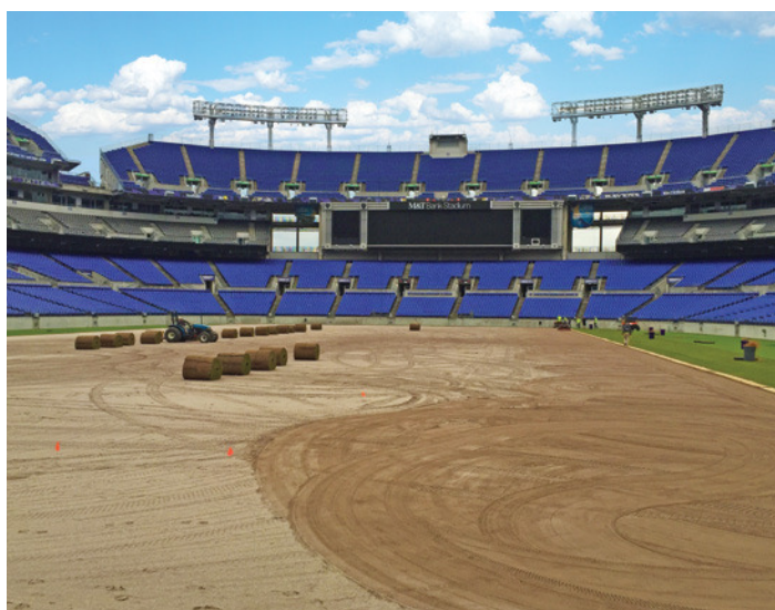
On the technical side, one key factor supporting the conversion from synthetic turf to natural grass at Baltimore’s M&T Bank Stadium was the team’s success in growing healthy turfgrass on three practice fields with Profile Porous Ceramic (PPC) Greens Grade inorganic soil amendments incorporated into the rootzone.
