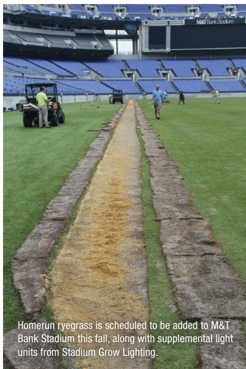
The Motz Group workers dug out 6 to 8 inches of crushed rock at M&T Bank Stadium — as well as the old rootzone — to reach the gravel layer, including the drain tiles and underground heating system that keep the field playable even in wet and freezing weather. The new 12-inch root zone, consisting of 90 percent sand, 5 percent native soil and 5 percent peat, was built on top of the existing gravel blanket.
