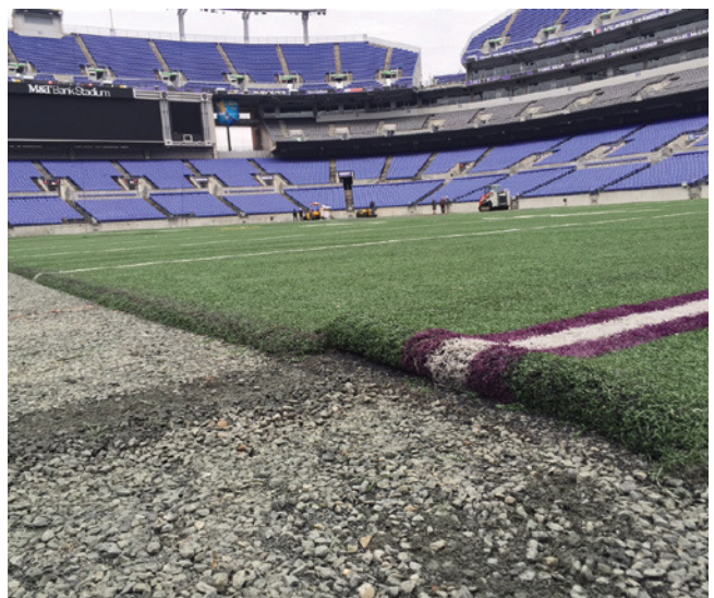
The Motz Group workers dug out 6 to 8 inches of crushed rock at M&T Bank Stadium — as well as the old rootzone — to reach the gravel layer, including the drain tiles and underground heating system that keep the field playable even in wet and freezing weather. The new 12-inch root zone, consisting of 90 percent sand, 5 percent native soil and 5 percent peat, was built on top of the existing gravel blanket.
