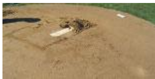
Outline your landing areas and plateau using a mound gauge to obtain the desired slope. Excavate 3" below the surface. Level and tamp firm.
