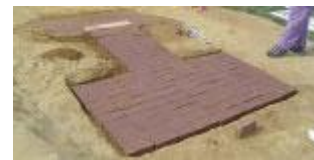
Wedge the blocks into position 1/2" below the rubber.
