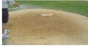
To repair holes, cut up blocks or use Professional Mound Clay. Before repairing, sweep out hole to expose pure packing clay. Moisten exposed packing clay, then add repair clay.
