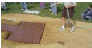
Tamp and water thoroughly several times for about an hour. Allow water to be absorbed into clay so blocks swell. Tamp firmly between watering.
