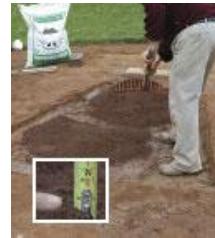
STEP 3: Evenly add an inch of new Turface Professional Mound Clay to the area you are working. Tamp until firm. Water the area, but do not drown. Repeat. As you near the last layer, reduce the amount of water you add to the Turface Professional Mound Clay.
