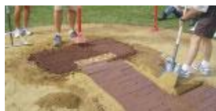
Fill around blocks with adjacent soil and tamp to wedge together.
